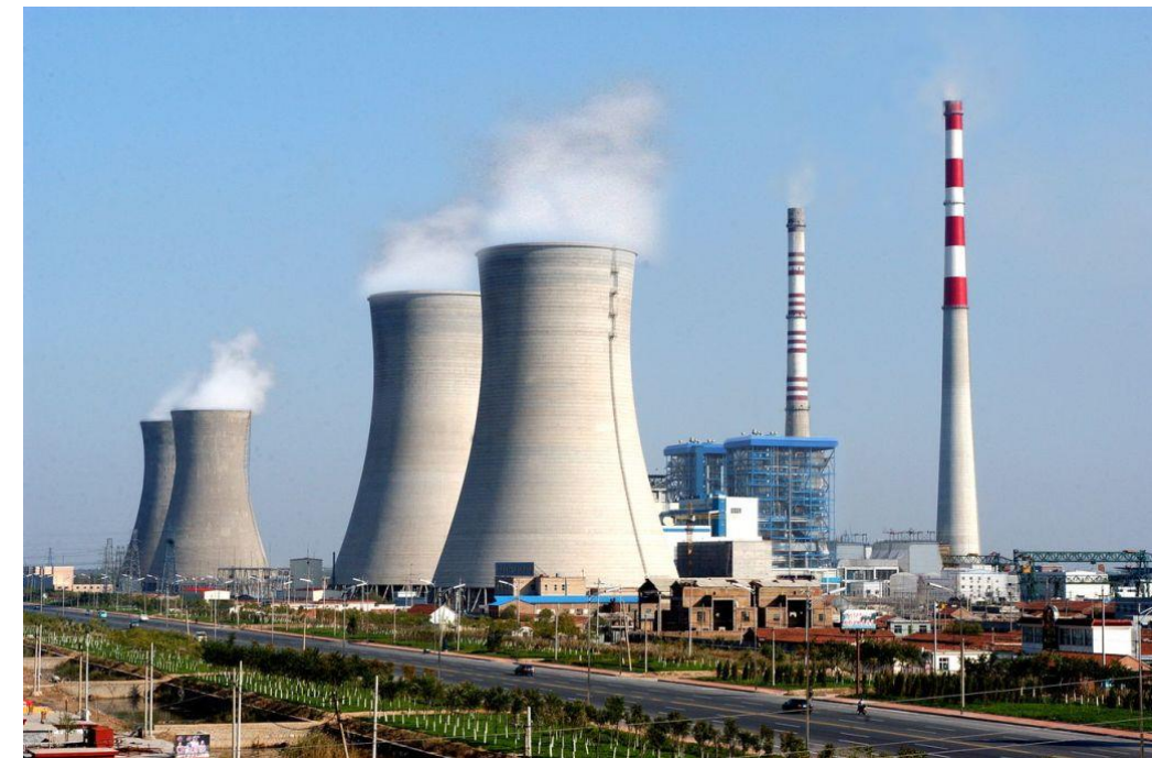
Fossil-fueled vapor power plant
